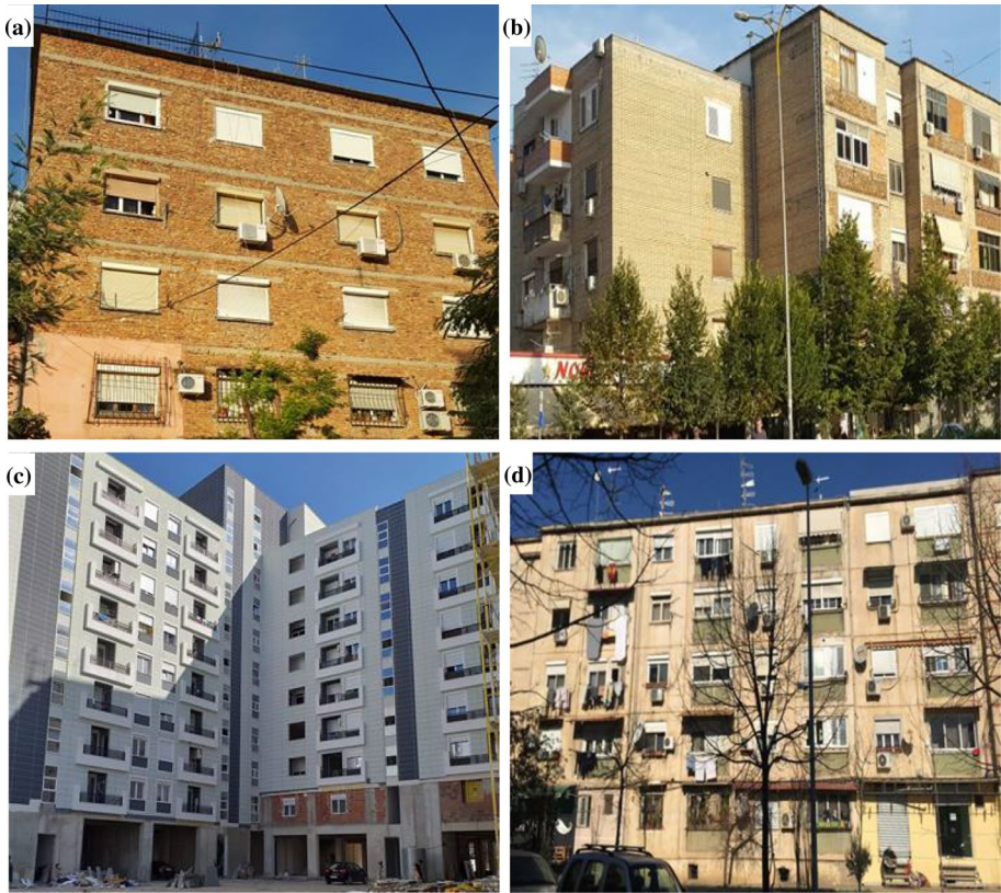
Fig. 5 Representative typologies of the multi-storey Albanian building stock: a unreinforced masonry building (URM) in clay bricks; b confined masonry (CM) building in silicate bricks; c new reinforced concrete (RC) building (under construction); d prefabricated large-panel building
