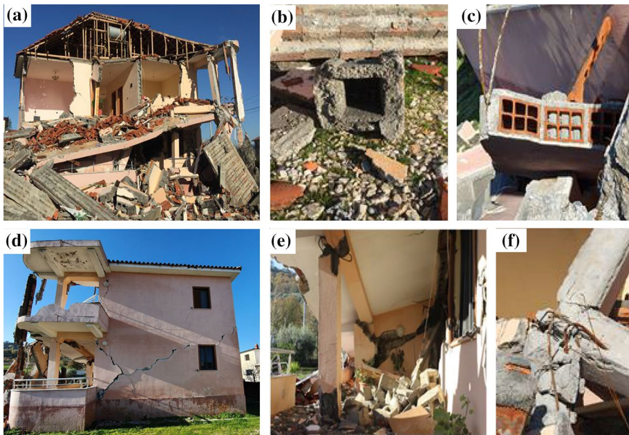
Fig. 9 Single-family rural houses in Bubq. a Failure of the front part of the building due to the collapse of the portico porch, b hollow concrete blocks of the bearing walls, c detailing of the hollow core prefabricated concrete slab, d severe crack of the rear building's façade due to the failure of the portico porch, e internal view of the portico porch, f details of the joint failure due to poor smooth reinforcements, which are completely corroded
