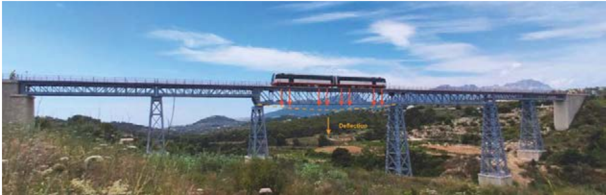
Figure 4: Static and load test on the bridge.
