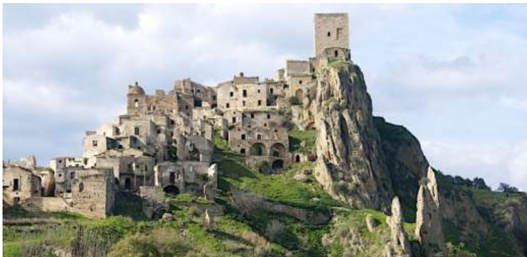
Figure 1. Medieval tower at the upper area of Craco (Matera, Italy).
