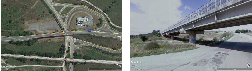
Figure 2.18: Google Earth data on the case-study B6 (top view from Google Earth and Google Street View image)
