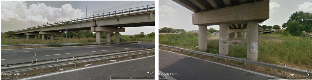
Figure 2.5: Street-view imagery for a case-study bridge
