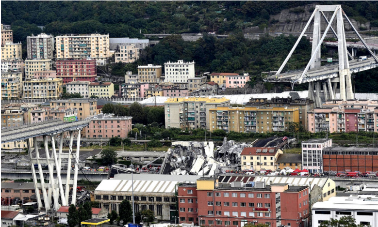
Figure 1.1: Collapse of the Polcevera bridge in Genova (Italy), 14th August 2018
