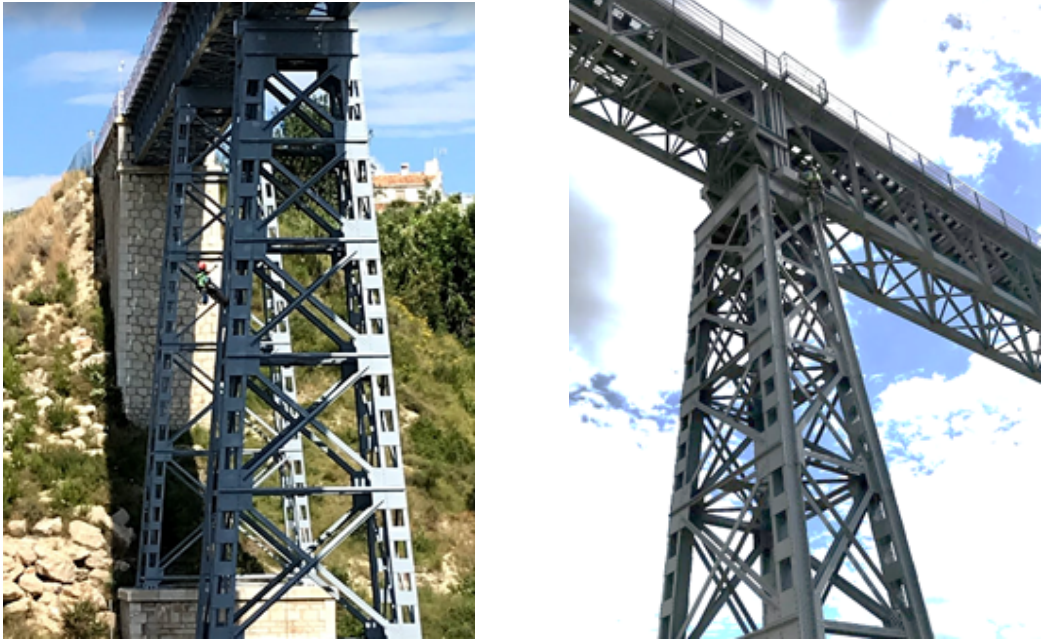
Figure 4.2: On-site photographs of riveted steel braced towers
