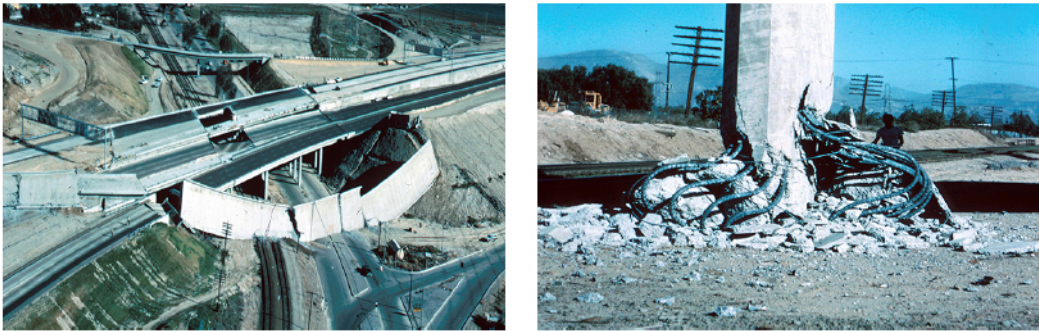
Figure 1.5: Damages on highway bridges, San Fernando earthquake, 1971 https://www.nbclosangeles.com/news/earthquakes/1971-sylmar-san-fernando-earthquake-california/3104/
