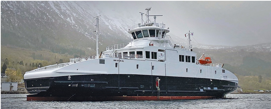
Figure 6.1: The ferry currently powered by batteries and diesel genset, chosen as a case study.
