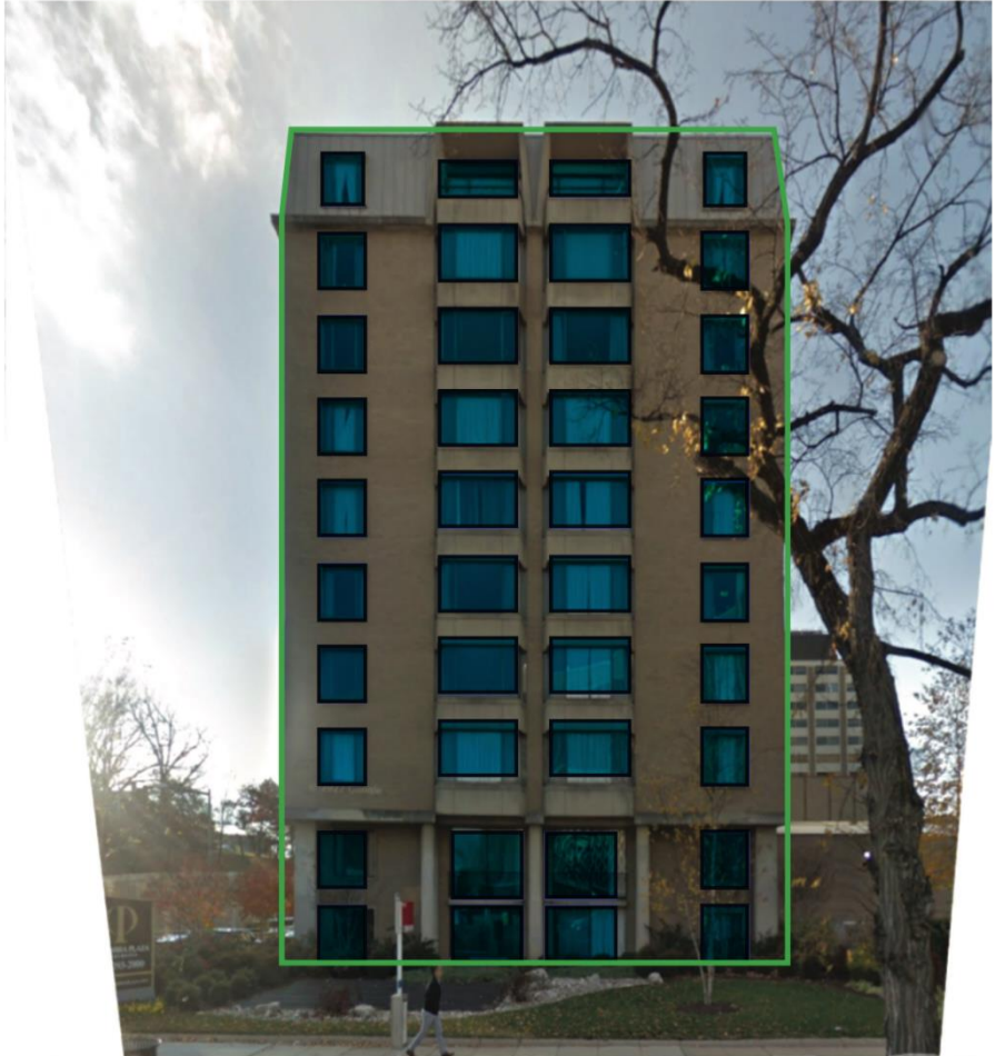
Figure 7 - Example of façade perspective rectification and WWR computation from Google Street View imagery. Data source: Google Street View API (2025); rectification via OpenCV; plot generated in Python/Matplotlib on 03-10-2025
