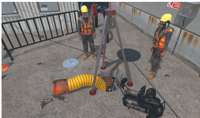
Fig. 5. The entry space of the underground utility compartment –Class A environment.
