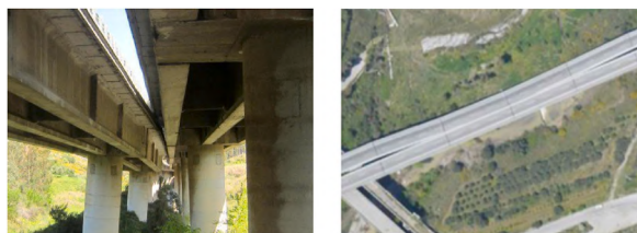
Fig. 1. The Himera viaduct in Sicily [10].
