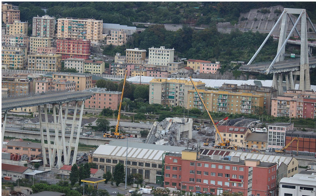
Fig. 1 - Collapse of the Polcevera bridge in Genova (Italy), 14th August 2018, (Sbarbaro, 2018).
