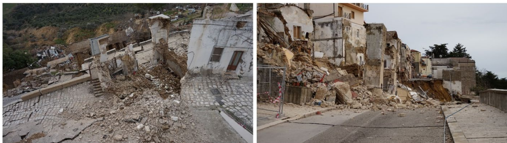
Fig. 64 - Observed damages on buildings and roads.
