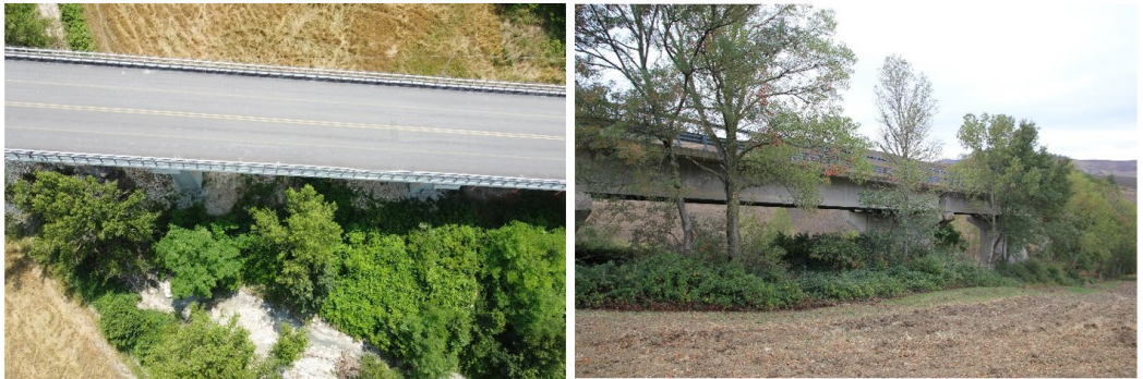
Fig. 69 - Photos of the focused existing bridge, reporting comprising a partial aerial view (left) and a lateral shot (right).
