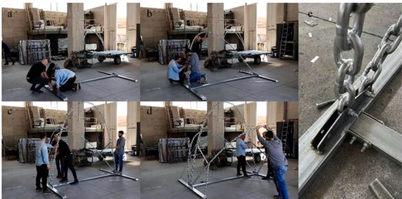
Fig. 9. The assembly phases of the metallic frame: a) assembly of the base; b) placement of the first arch; c) placement of the second arch; d) placement of the third arch; e) a detail of the assembly system.
