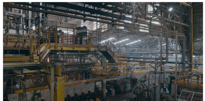
Fig. 2. Case of study: hollow glass industry, glass plant in south Italy.
