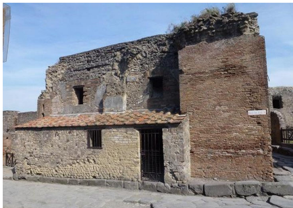
Figure 1. Main entrance of the Forum Women's Thermal Baths building.
